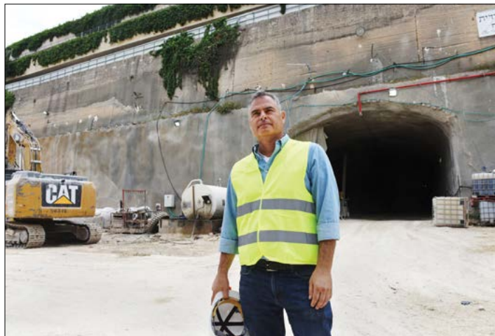
Arik Glazer, managing director of Rolzur, stands outside one of the tunnel entrances to the underground cemetery project.
